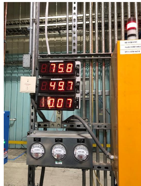
Figure 6: Booth Monitoring Stack Showing 75.8°F and 49.7% RH
